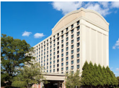
Sonesta Atlanta Airport North 378 Rooms 17 Meeting Rooms Largest Space 4,050 sq. ft.
